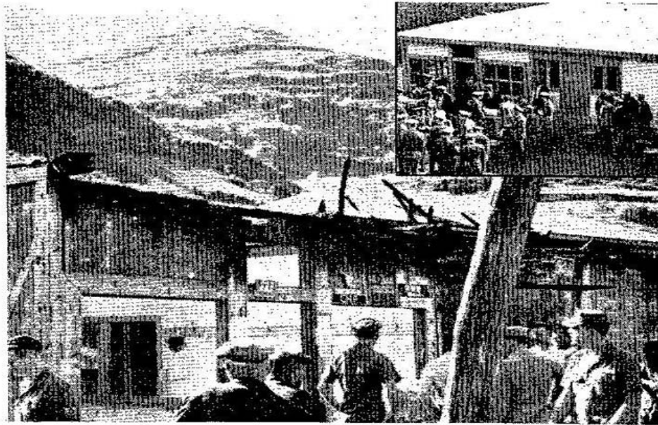
A HAND —The burned out shell of an elderly native's combination tea house-home is surveyed by members of TUSLOG DET 3-1 prior to their pitching in to rebuild the establishment as a symbol of their good will. Keys to the new home (insert) were presented to the grateful owner in recent ceremonies. (Photos by A. R. Johnson)
